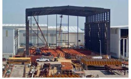
Carpenter Wright Engineers a division of Bennett & Pless Structural Carpenter Wright Engineers and VP Buildings provided the structural design for the approximately 42,300 SF, 80 foot tall, hybrid structural steel and preengineered building for the assembly of ship engines for Northrup Grumman Ship Systems.
