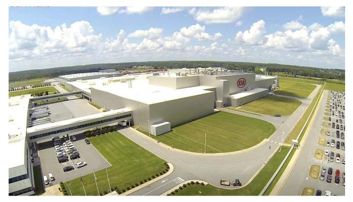
Bennett & Pless Structural Originally designed in South Korea, B&P became the Structural Engineer of Record for the 2 million square foot facility. As the EOR B&P provided review and redesign of the assembly plant, welding and stamp buildings. The facility is the first manufacturing site in North America for KIA Motors. With an annual capacity of more than 340,000 vehicles, this facility represents a \$1.1 billion investment on 2,200 acres.
