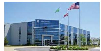
The new 300,000 SF advanced manufacturing plant produces precision, super-alloy machined parts for GE jet engines. Features included 280,000 SF shell production space, 24,000 SF two-story office space, utility/process piping and equipment, centralized compressed air system, and a centralized cooling tower system.
