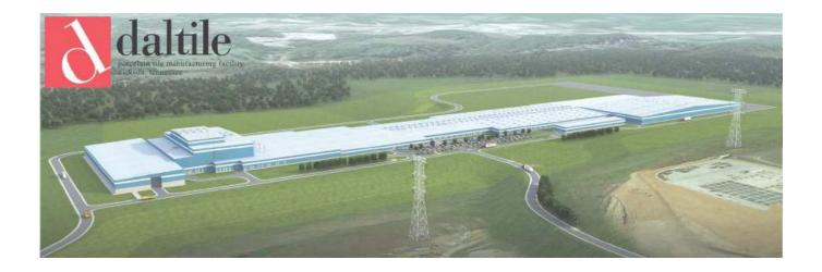
Carpenter Wright Engineers a division of Bennett & Pless Structural I. C. Thomasson Associates Mechanical Design Architectural, structural, preliminary mechanical and project management services were provided for a new 1.2 million SF porcelain tile manufacturing facility (shell only). Six primary functional areas of the facility are raw material storage, body prep and spray drying, glazing, kiln, packing, and warehouse storage.
