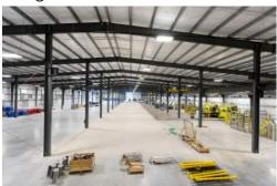
The TIS team provided full planning and design services, including architectural, site/civil, structural, mechanical, electrical, plumbing and fire protection design services for a new 115,000 SF light manufacturing (pickling, drawing, stranding of structural wire) and warehouse facility with interior office and employee amenities area. The construction is a Pre-Engineered Metal Building (PEMB) structure.
