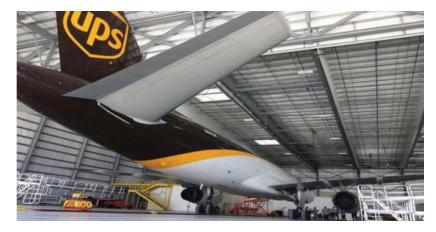
CWE designed the two-span box truss structure to support the pre-engineering building frames to construct a 530,000 SF aircraft maintenance and repair hangar at the Pensacola International Airport. The box truss was approximately 27 feet deep, and was designed for 2 spans of approximately 300 feet each. At the mid-span of each of the 300 foot spans, a notch in the bottom of the box truss was created for the tail of an aircraft. The clear height under the box truss was 51 feet.
