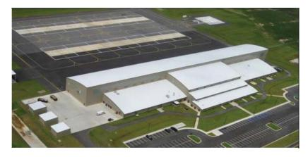
CWE provided structural design of the three 240 foot long box trusses and support trusses for the mega-doors for the military helicopter hangar, and the roof trusses and support columns for the juncture of the curved roof girders at the building height transition. Each box truss was designed for two spans of 120 foot each. The area of the helicopter hangar was approximately 80,000 SF. The facility includes numerous under-hung frames to service the aircraft.
