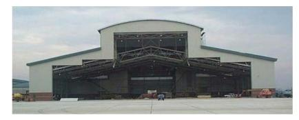
Carpenter Wright Engineers provided the structural design for the approximately 80,000 square feet C-5 Corrosion Control Hangar facility. The corrosion control hangar facility consists of a high hangar bay for a C-5 aircraft and a lower bay for maintenance shops.
